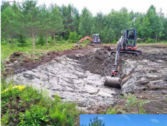
Above: Excavating the first half of the pond
